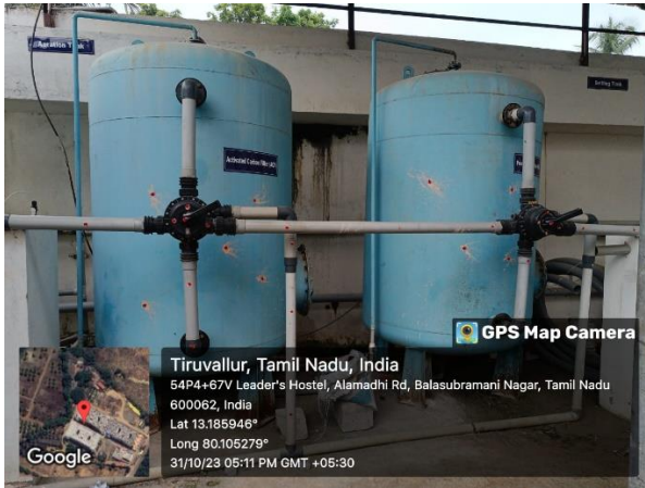
Fig- 6. Sand Filter and Activated Carbon Filter
