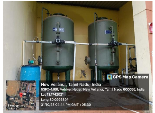
Fig- 6. Sand Filter and Activated Carbon Filter
